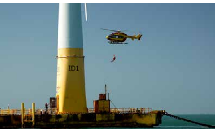
Helicopter exercise on the Floatgen wind turbine (March 2022)
